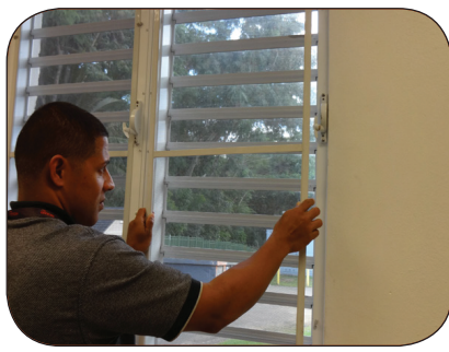
Install or repair window & door screens.
